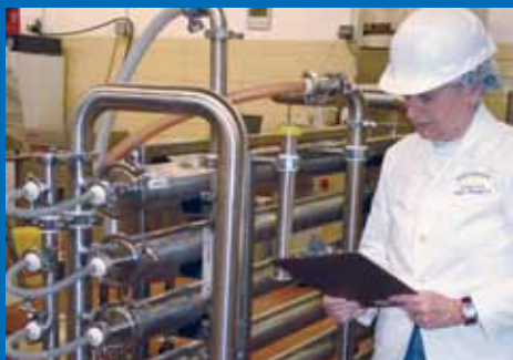
Membrane filtration equipment at the WCDR.
